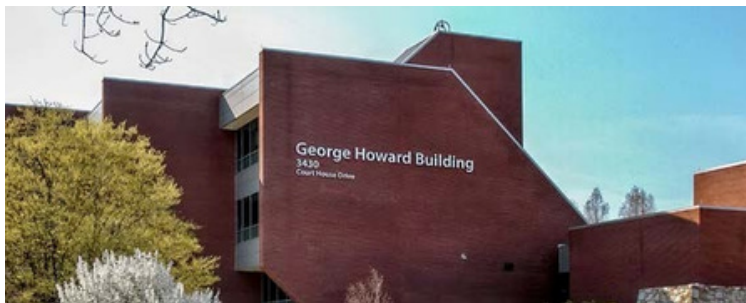
GEORGE HOWARD BUILDING · HOWARD COUNTY, MARYLAND
